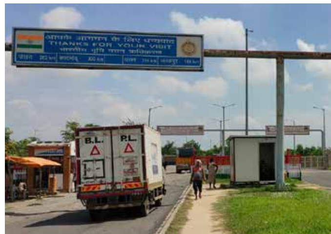
Raxaul Land Port: Road connectivity
