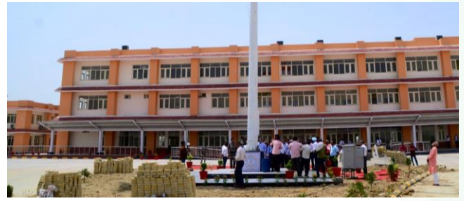
Rupaidiha land port's construction nearing completion.
