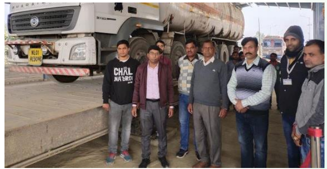
The newly installed weighbridge at the import shed at Jogbani land port.
